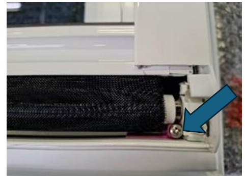
Figure 6 The pre-drilled screw holes that are located under the covers. The arrow points to one of these holes.
