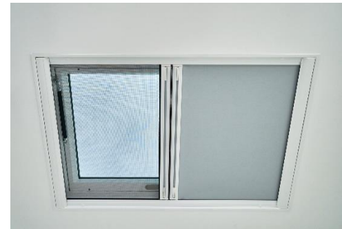
Figure 11 Double roller blind of our roof window
