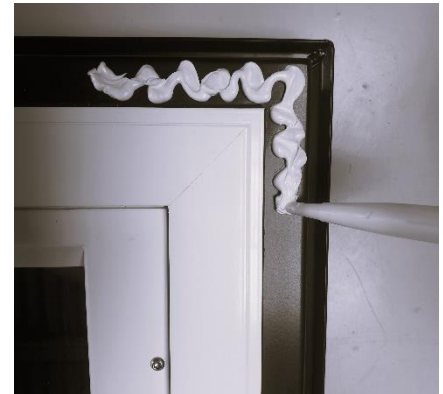
Figure 3 Applying glue to the built-in frame.
