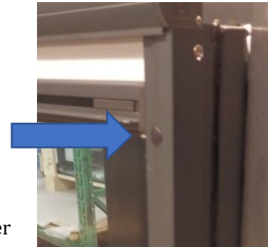
Figure 5 Double roller blind model B. The arrow points to one of the covers that you can open.
