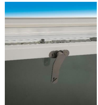
Figure 9 The roof window in ventilation position.
