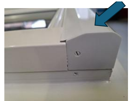
Figure 6 The pre-drilled screw holes that are located under the covers. The arrow points to one of these holes.
