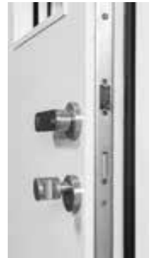
Figure 7 Side view of the inside of the door, with locking button.
