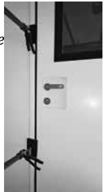
Figure 5 The door is fixed to the wall using supports, this is an example but can also be done with adhesive tape.
