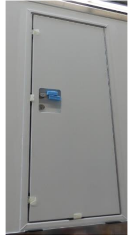
Figure 4 Spacers to keep the door in the right position during installation.
