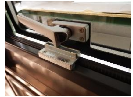
Figure 10 The stainless steel handle with the black locking button.
