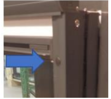
Figure 7 The arrow points to one of the predrilled holes.
